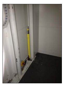
4. Depending on entrance, locate rod in either hole on yellow tab and lever up. PP should then drop down under its own weight. **The PP is now activated.**
